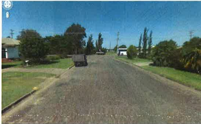
Partridge Street, looking east to the East Street Intersection
